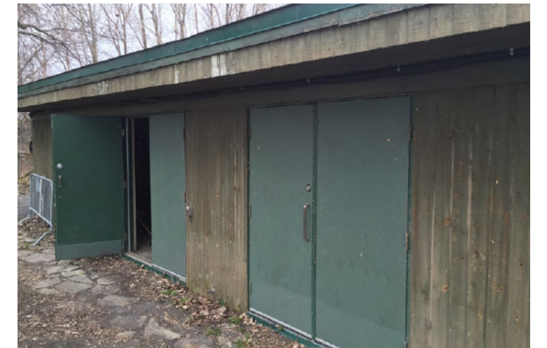
Station d'épuration, Jonathan Cha, 2016.
