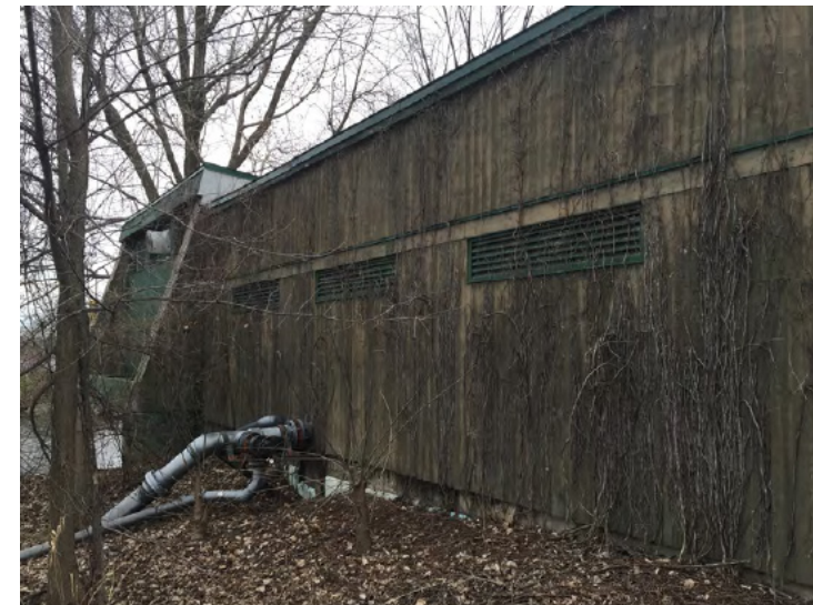
Station d'épuration, Jonathan Cha, 2016.
