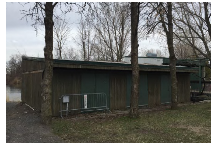
Station d'épuration, Jonathan Cha, 2016.
